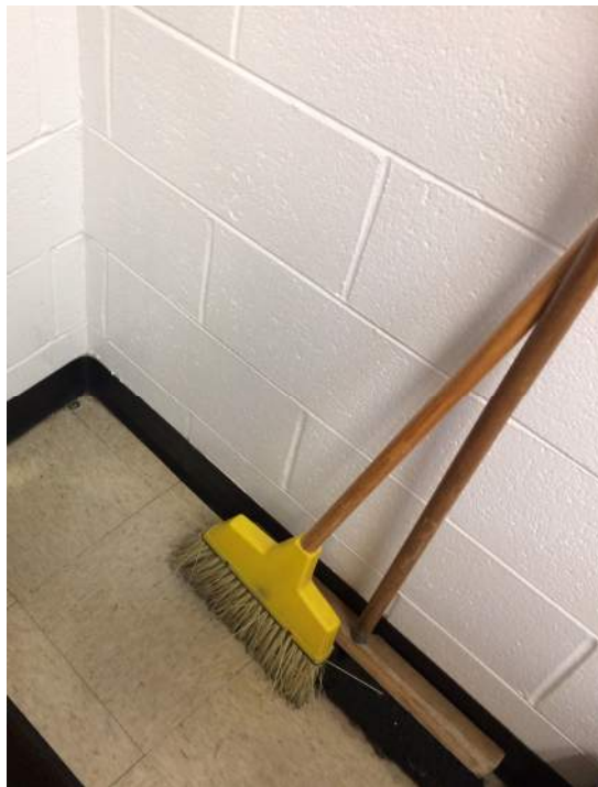
Photo 27: View of Homogenous Area 27 FMS Room 105
