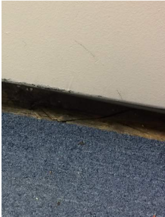
Photo 13: View of Homogenous Area 13 Room 107
