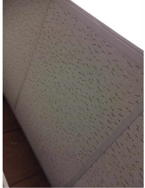
Photo 14: View of Homogenous Area 14 Room 107
