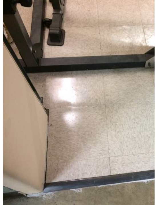
Photo 6: View of Homogenous Area 6 Room 102
