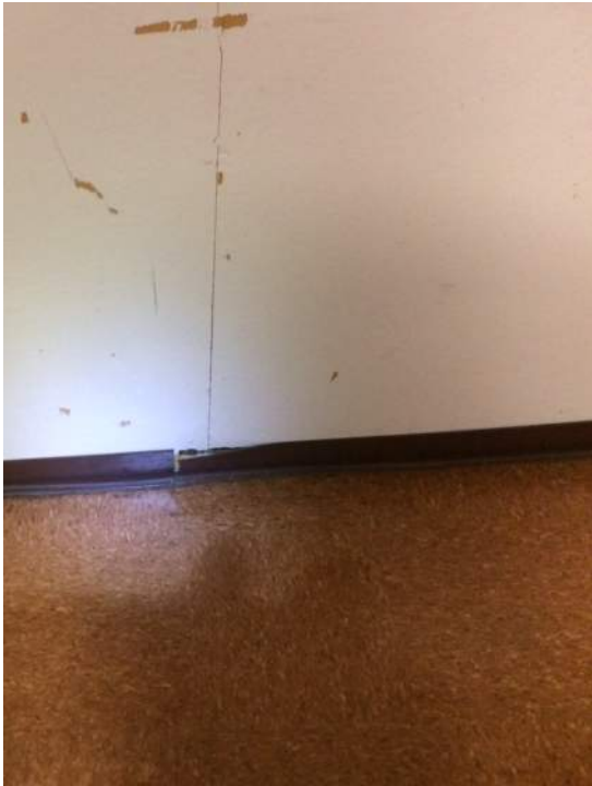
Photo 25: View of Homogenous Area 25 Room 118
