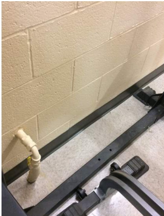
Photo 7: View of Homogenous Area 7 Room 102
