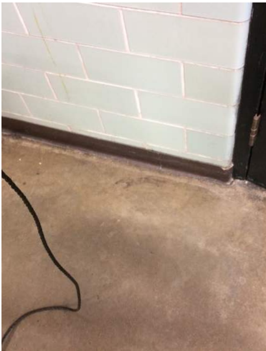
Photo 3: View of Homogenous Area 3 Room 101
