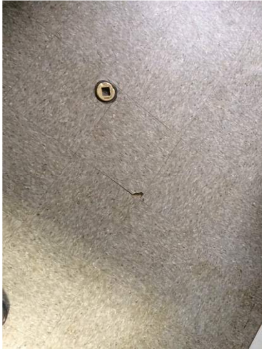
Photo 9: View of Homogenous Area 9 Room 131
