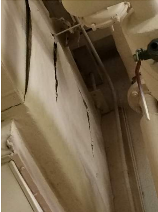
Photo 5: View of Homogenous Area 5 Room 101
