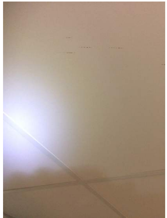
Photo 20: View of Homogenous Area 20 Room 125
