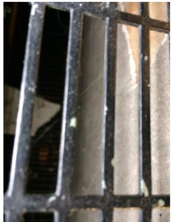
Photo 24: View of Homogenous Area 24 Room 123
