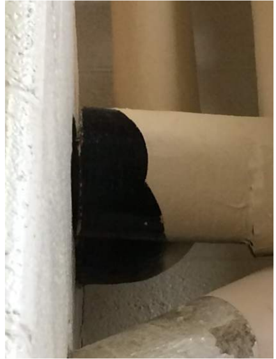
Photo 2: View of Homogenous Area 2 Room 101
