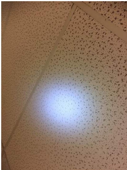
Photo 23: View of Homogenous Area 23 Room 123
