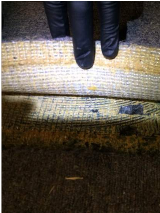
Photo 15: View of Homogenous Area 15 Room 112
