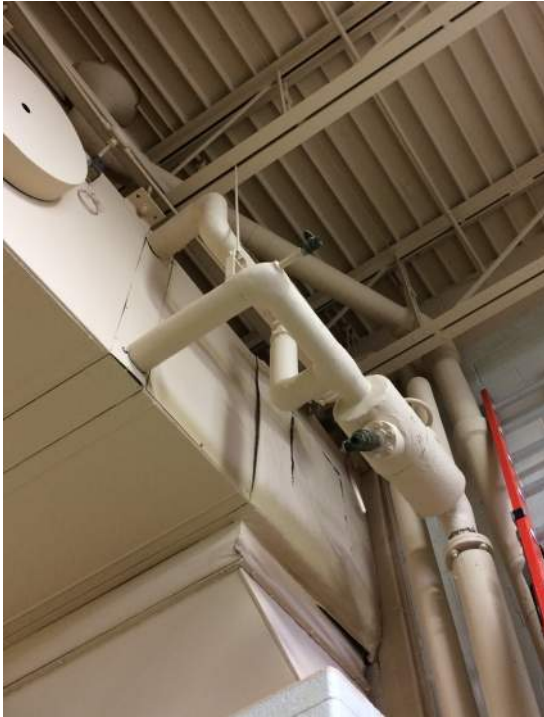
Photo 1: View of Homogenous Area 1 Room 101
