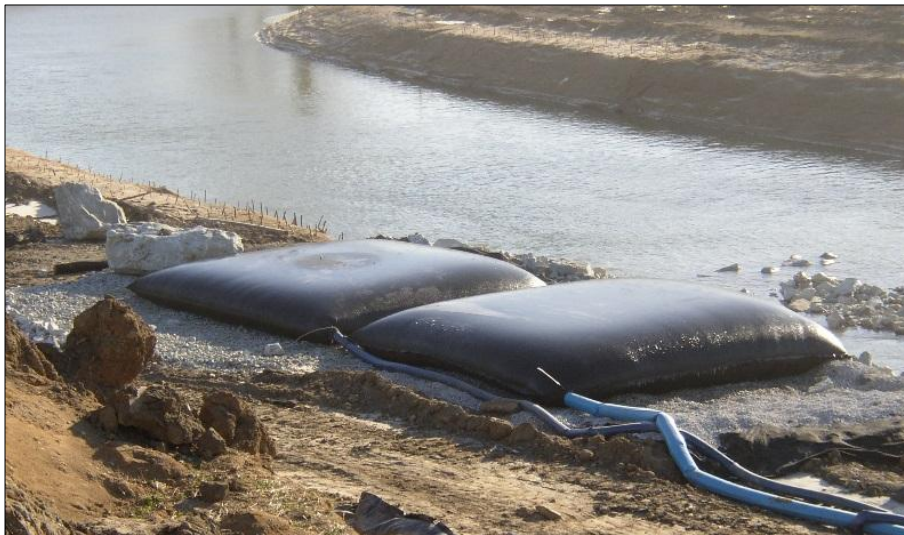
Exhibit 713.01-A. Filter bags installed on a level aggregate pad with a stabilized discharge or outflow path to the receiving stream.
