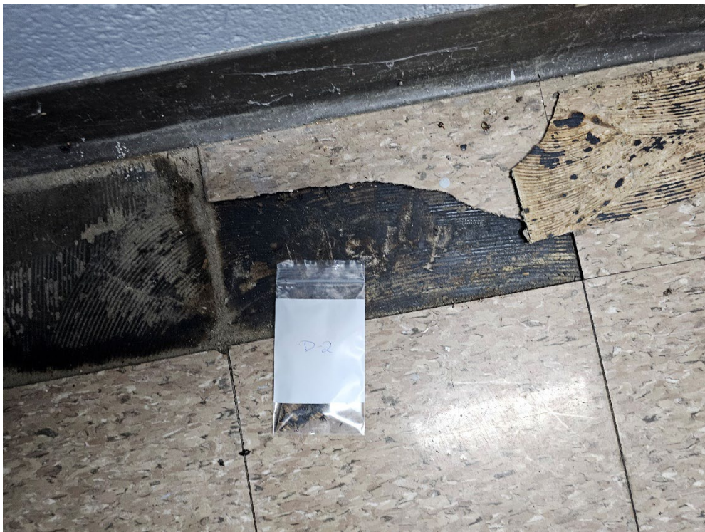
Photo 2: View asbestos-containing black mastic below office hallway floor tile (Sample D-2)
