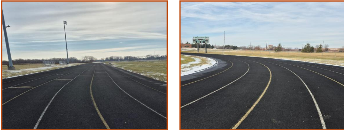
Figure 1 – Photographs Taken at the Time of our Field Investigation
