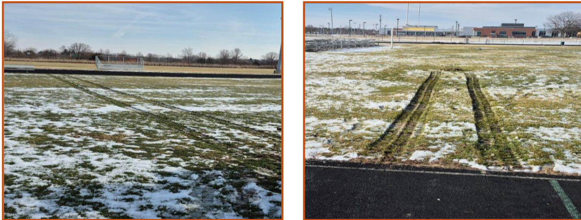
Figure 2 – Photographs of the Infield Surface After our Field Investigation
