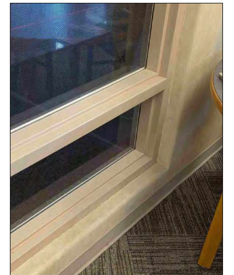
7 EXISTING WALL PAPER AT OPNG. SCALE: PHOTOGRAPH FOR REFERENCE
