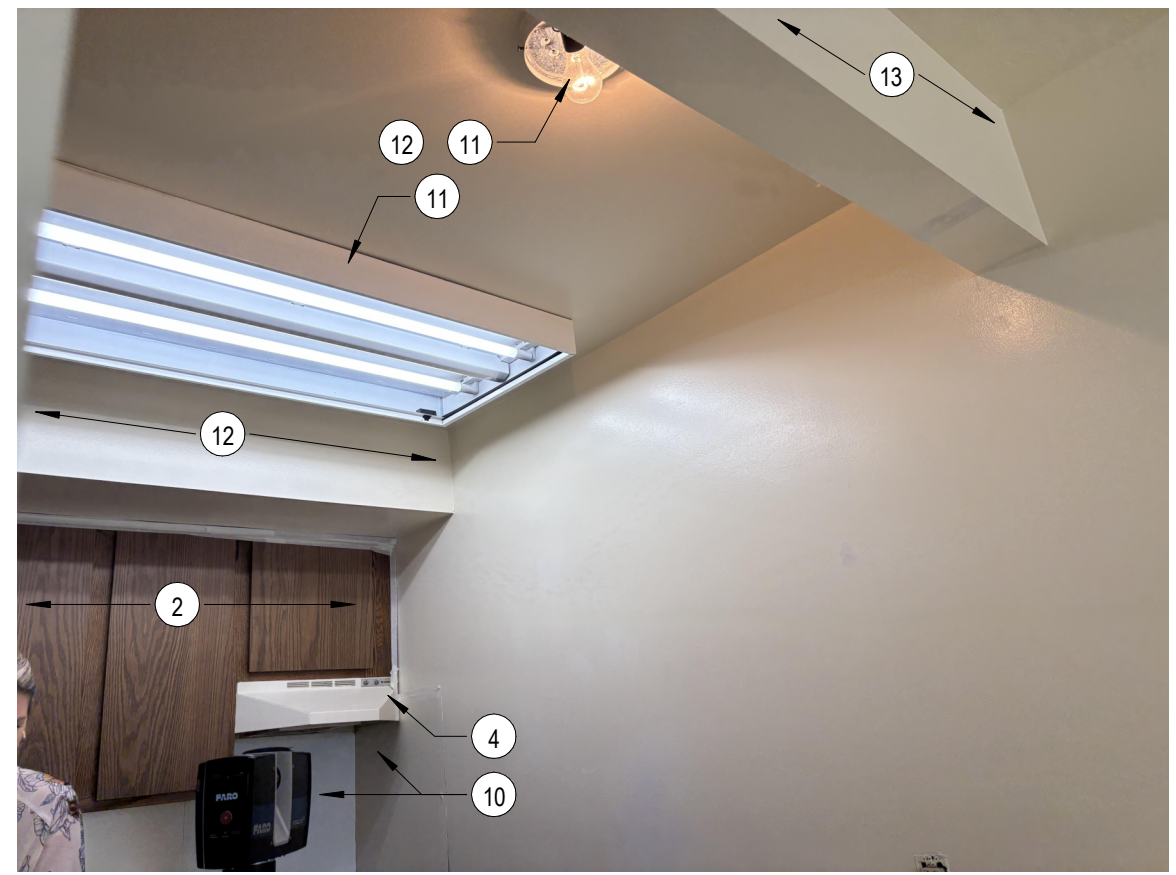
IMAGE 5 - 1ST FLOOR UNITS BULKHEAD
